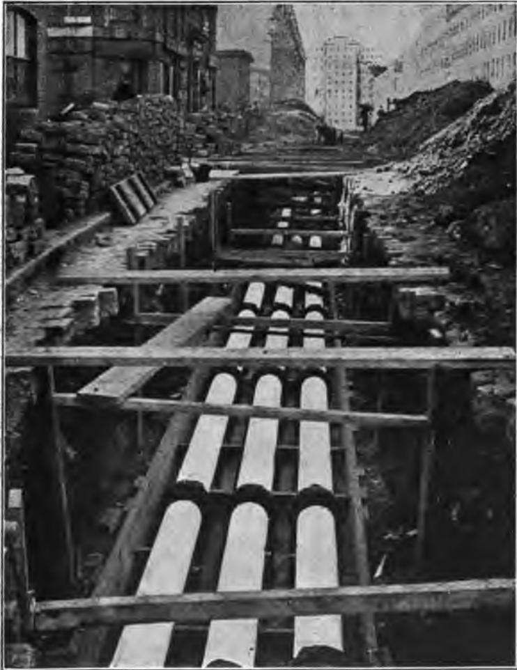
FIG. 265.—Three-pipe Brine System.
